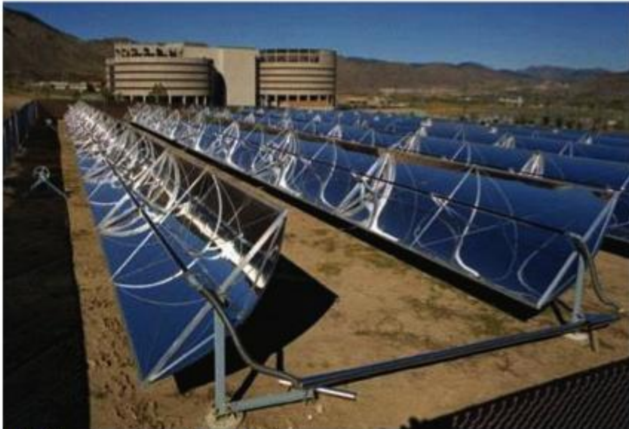
Parabolic trough concentrators. Source: NREL.
